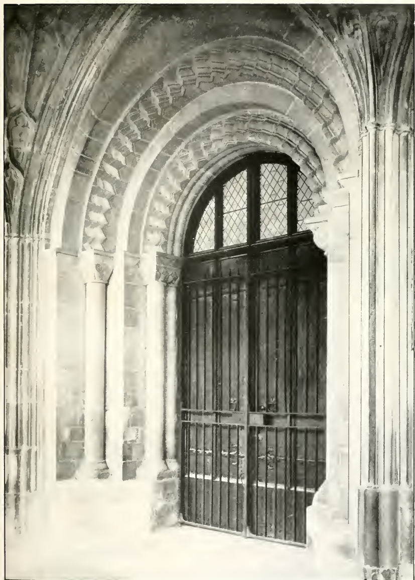
FIG. 4.—GLOUCESTERSHIRE CATHEDRAL, CHAPTER HOUSE DOORWAY.
